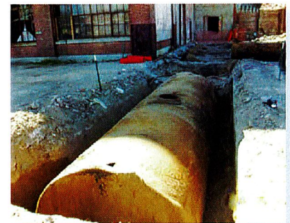
Multiple Underground Storage Tanks at Orchard Whitney Site
