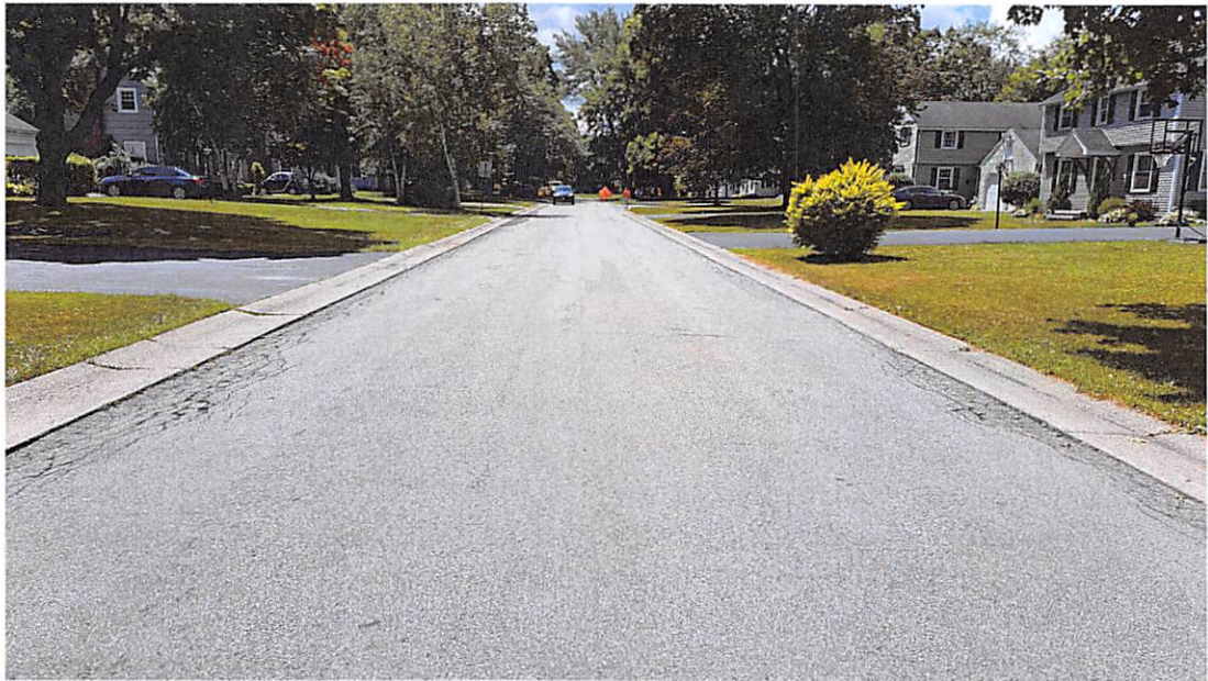
Image 1: Idlewood Road's 19ft wide asphalt roadway with concrete 'v' shaped gutters on either side. Would you drive down this road with two wheels in the gutter?
