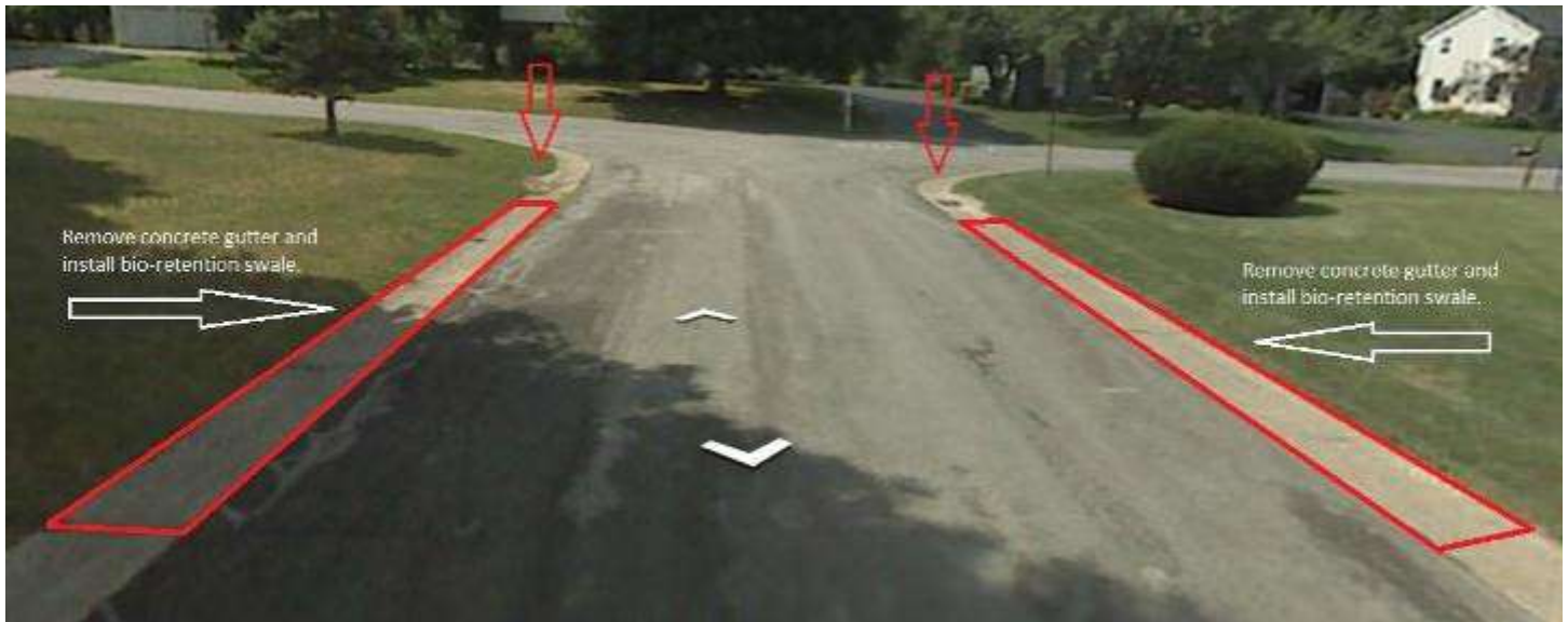
Figure 7: Above is an example typical residential street. Stormwater runoff is channeled into the concrete gutters along the sides of the road and conveyed to the stormwater sewer system through the storm inlets (red arrows). In order to reduce runoff into the stormwater sewer system and increase infiltration, bio-retention swales could be installed. These green infrastructure retrofits would replace the concrete gutter and contain stormwater runoff and allow it to infiltrate back into groundwater.
