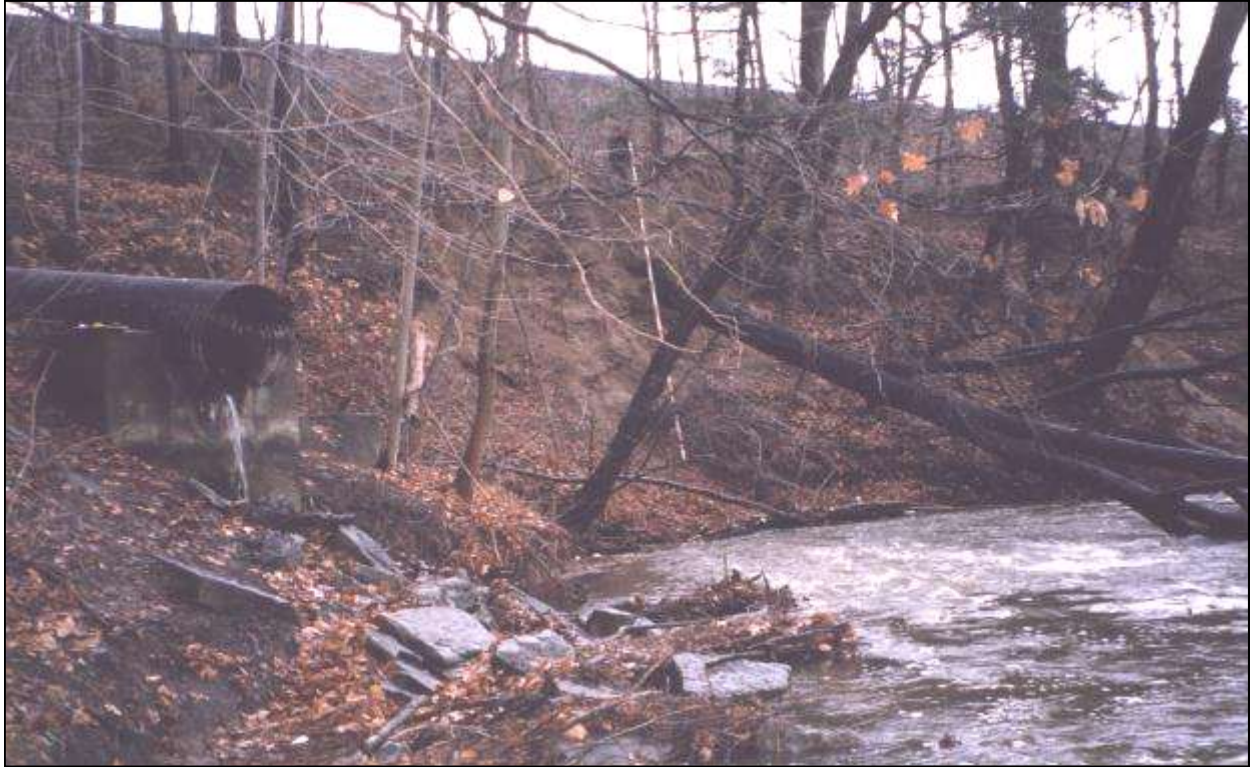
Figure 3: Severe streambank erosion above Corbett's Glen (note railroad embankment at top of bank)
