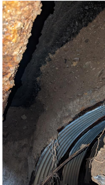
Utility and pavement undermining
