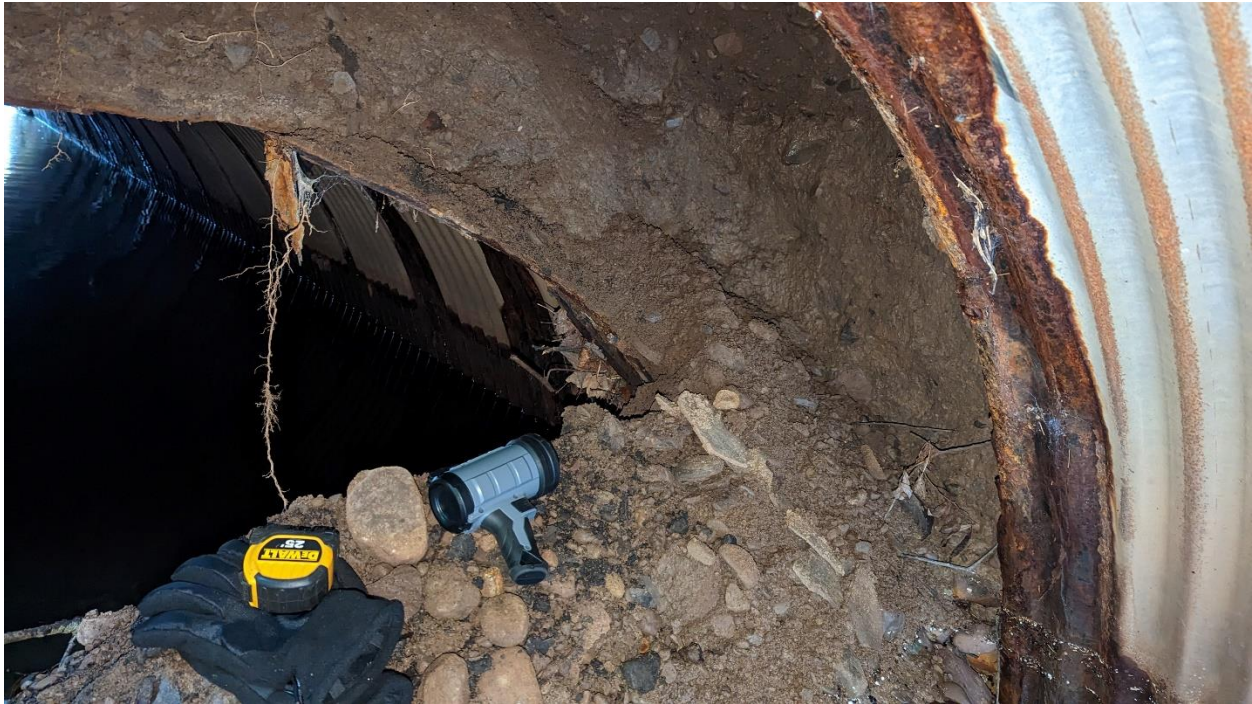
Cracked headwall at outlet end
