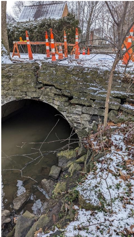
Cracked headwall at outlet end
