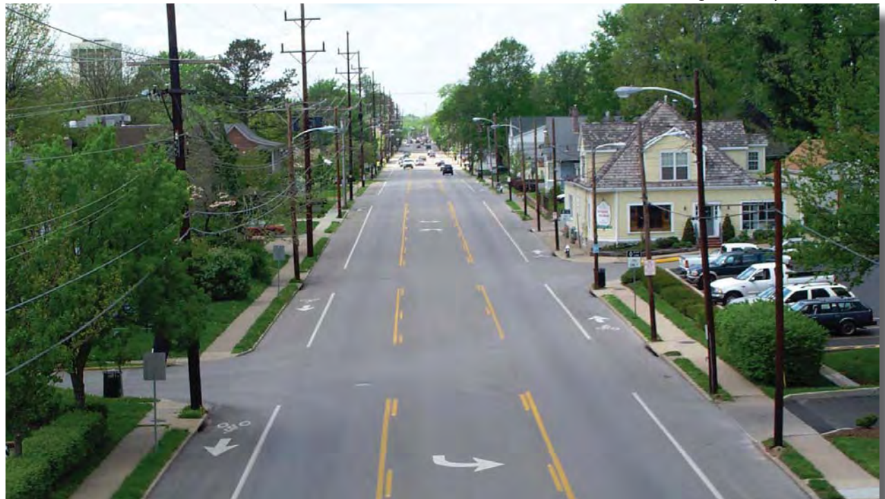
(Below) The same section of Euclid Ave. after "road diet" completion in August 2000. Source: ContextSensitiveSolutions.org Case Study #15
